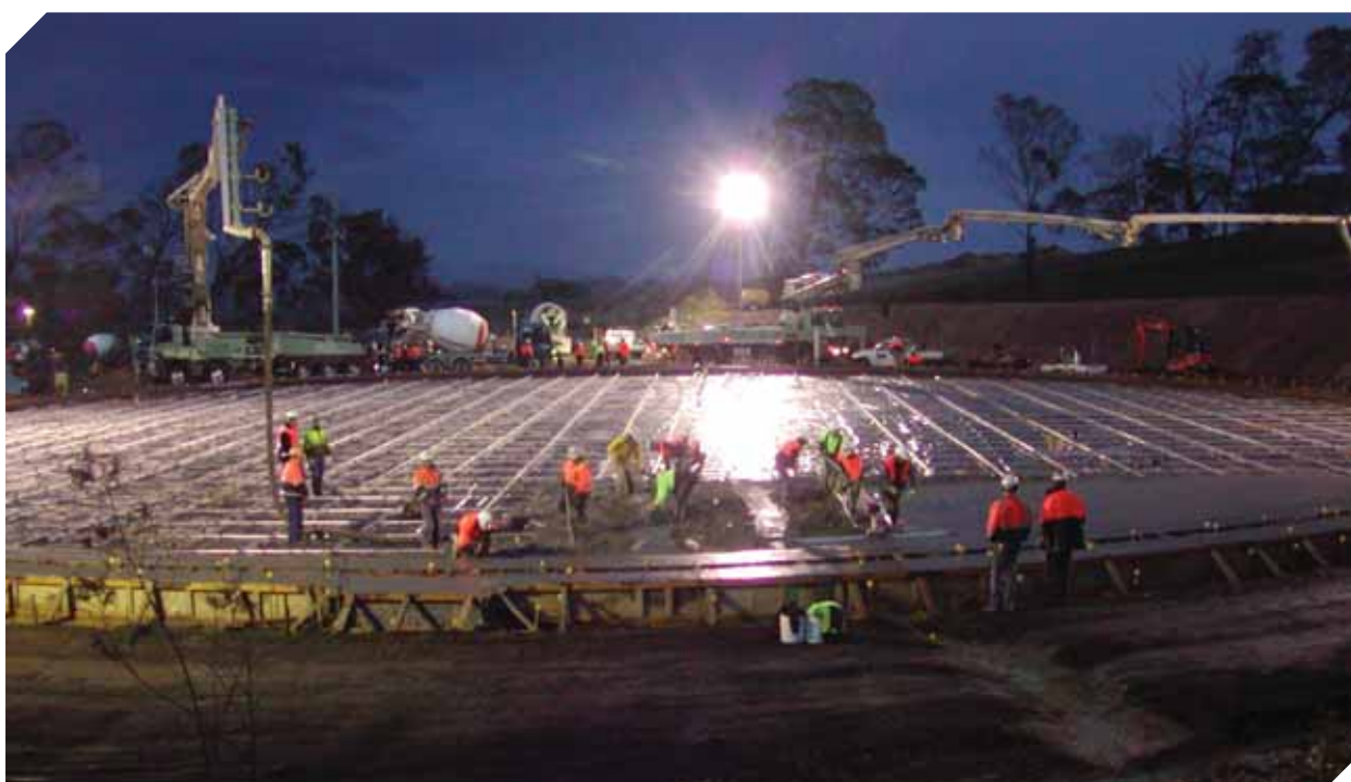
Concrete pour for the base of the new Kilmore water storage
