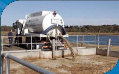
Trade Waste discharge at Broadford wastewater management facility
