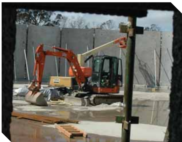
Construction of new Kilmore water storage
