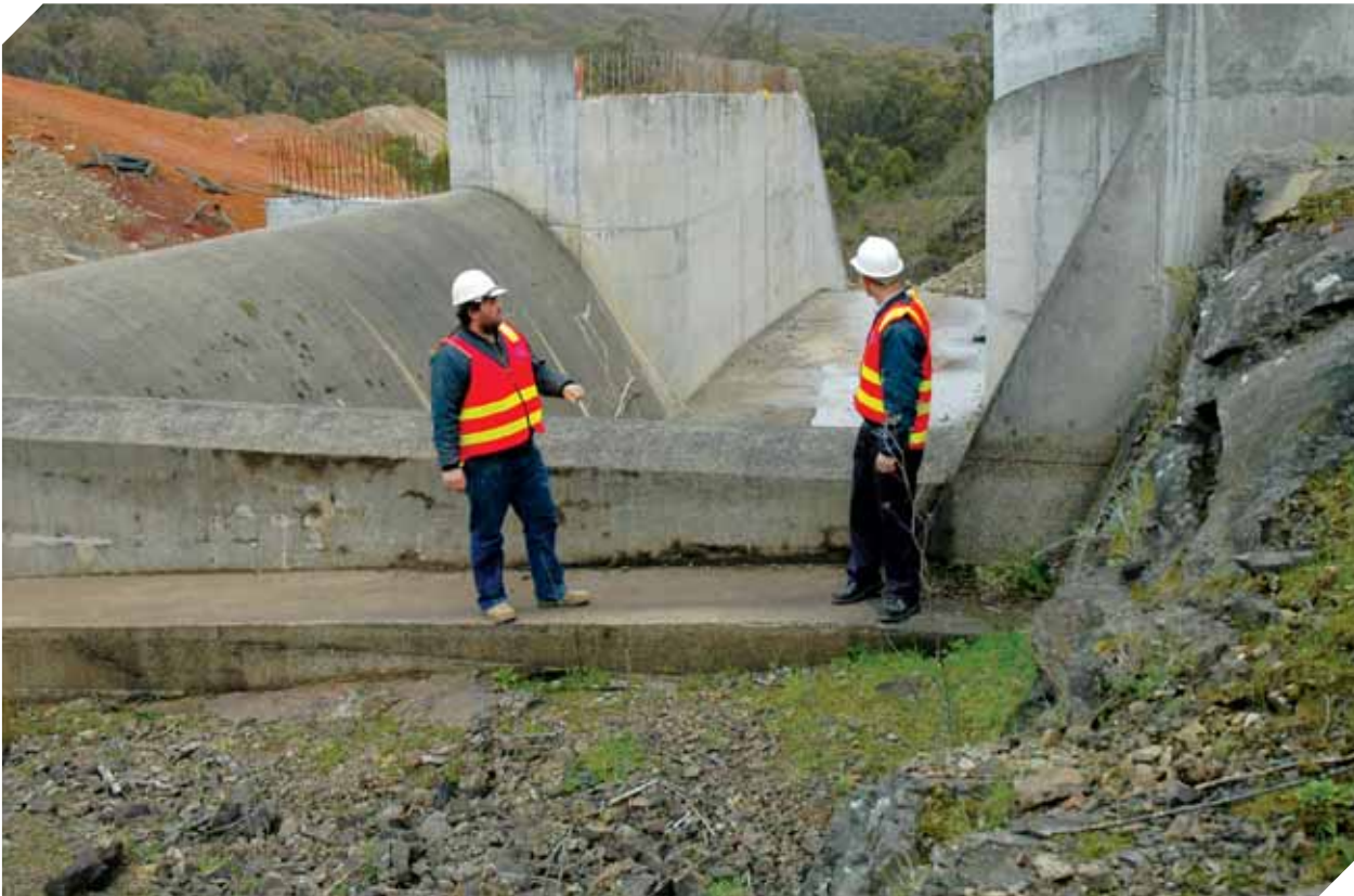
Adrian Voogt and Mark Putman at the Sunday Creek Spillway
